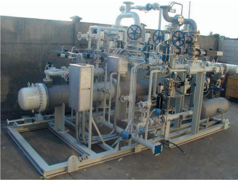
U.K. Application Power Plant Vacuum system
