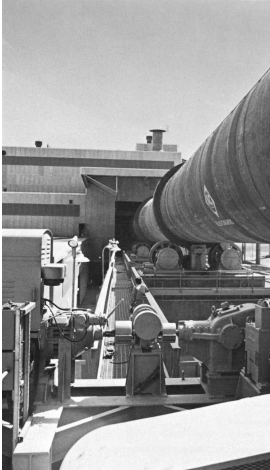
Photo: Marland CECON clutch and CEBMAG Backstop on modern cement kiln provide for emergency drive rotation in case of main power shutdown.
